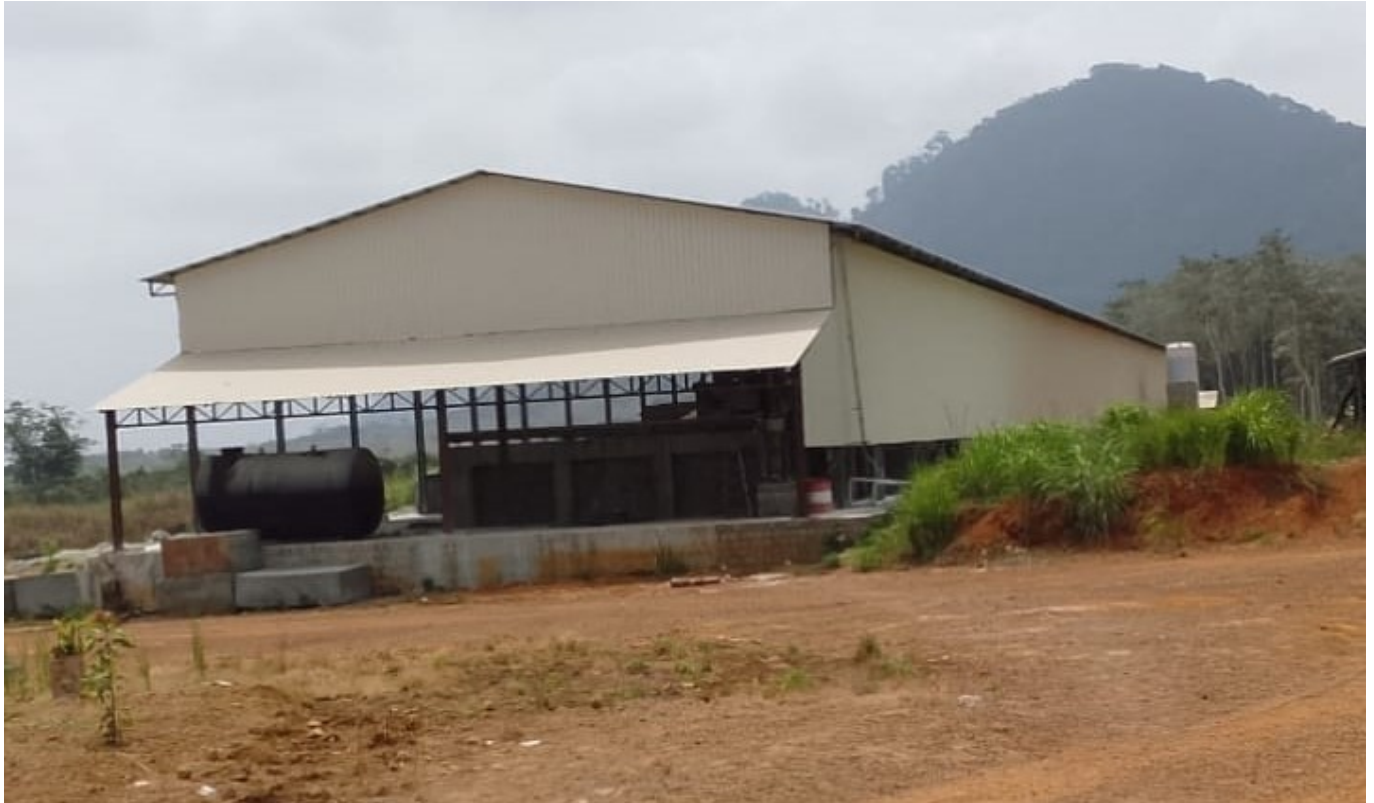
The plant of Tuolei Stone SL Limited in Gbonkoh Lal. Photo Credit: Jonathan Jackson Komeh.
